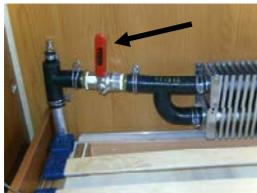
The convectors in the rear bed area and in the alcove (depending on floor plan) are connected to the heating circuit via a bypass which can therefore be regulated separately with the valve on the convector.
